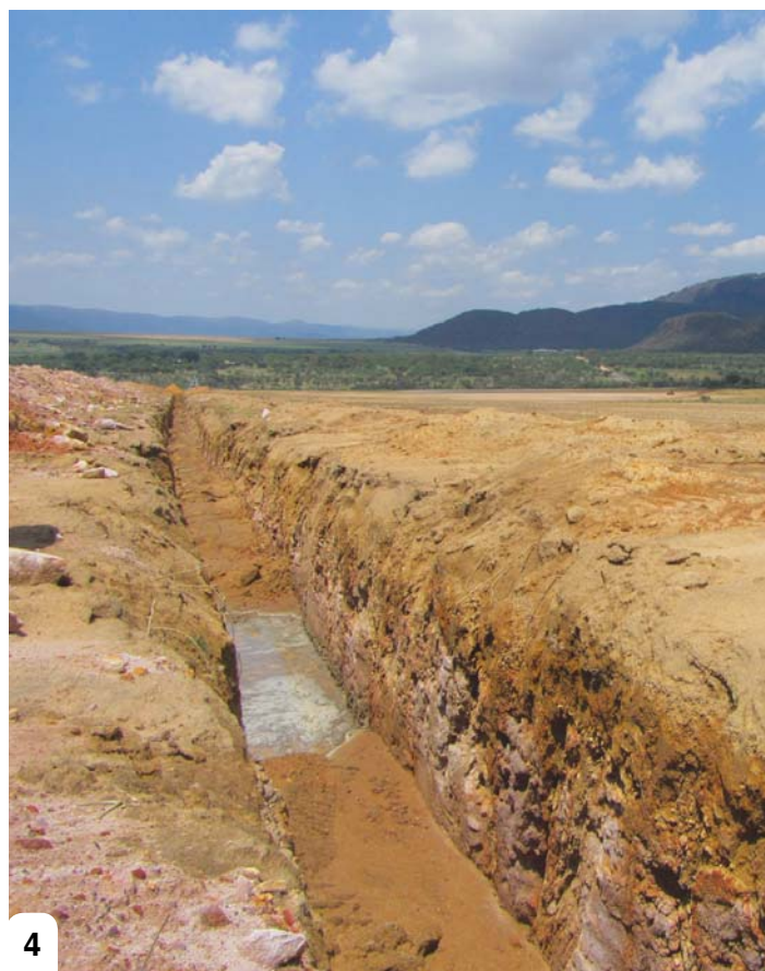
Subsurface drains are in the process of being installed.
