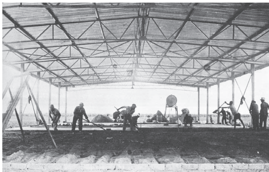
The first buildings on the permanent Harvest Day Grounds were erected in 1974 . Here the floor of one of the restaurants is poured.
