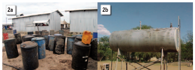
▲ 2a and 2b: Insufficient storage conditions of fuel include those in barrels exposed to rough elements of nature and also bulk storage tanks without filtration and breathers.
