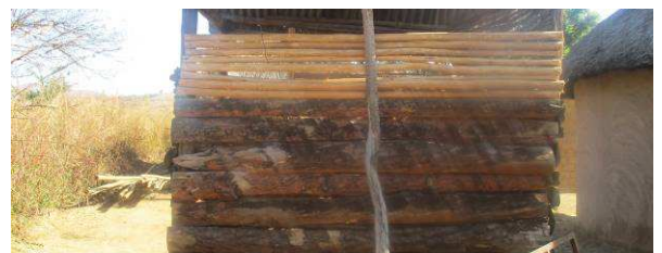
Neliwise Msele from Stuwlane constructed a new maize storage structure for her harvest.
